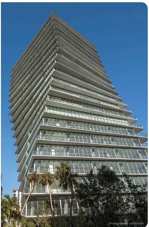
Custom-designed floor-to-ceiling windows made with Solarban® 72 glass and balcony railings laminated with Starphire® glass not only give Grove at Grand Bay "curve" appeal but also help protect against hurricane damage.
